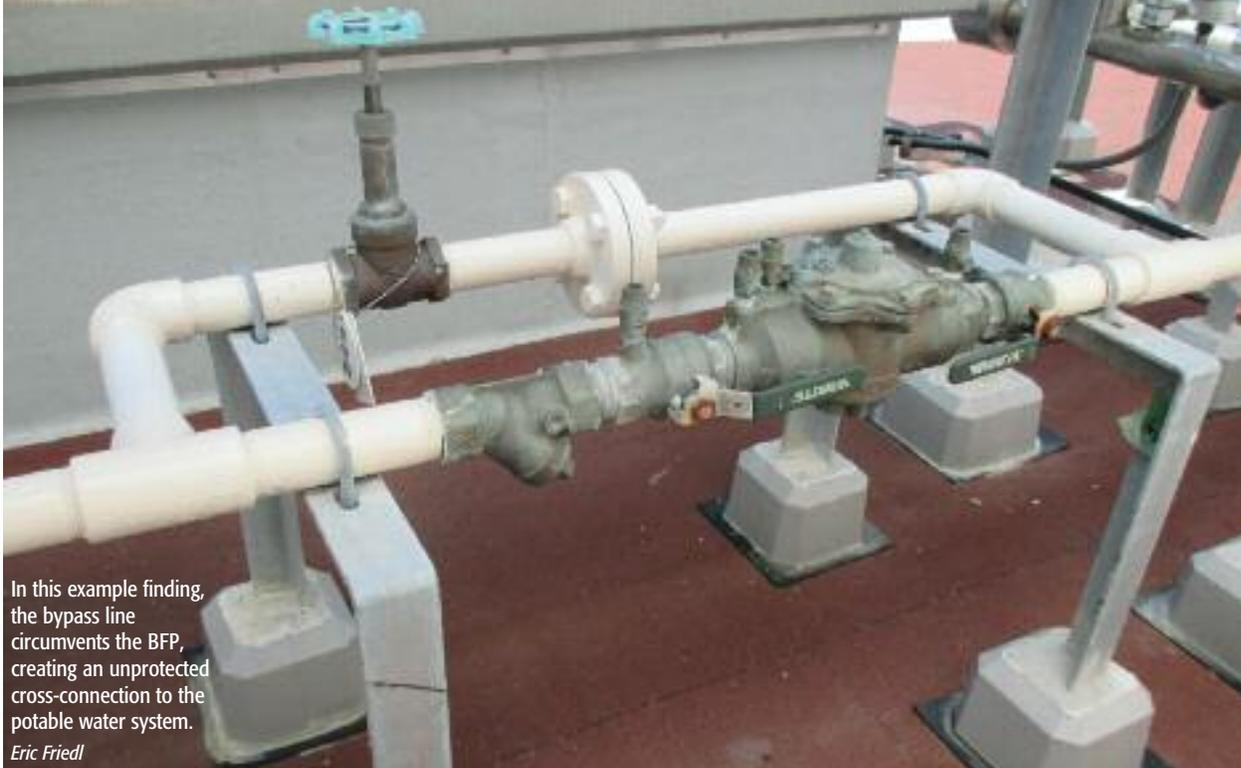
In this example finding, the bypass line circumvents the BFP, creating an unprotected cross-connection to the potable water system.
