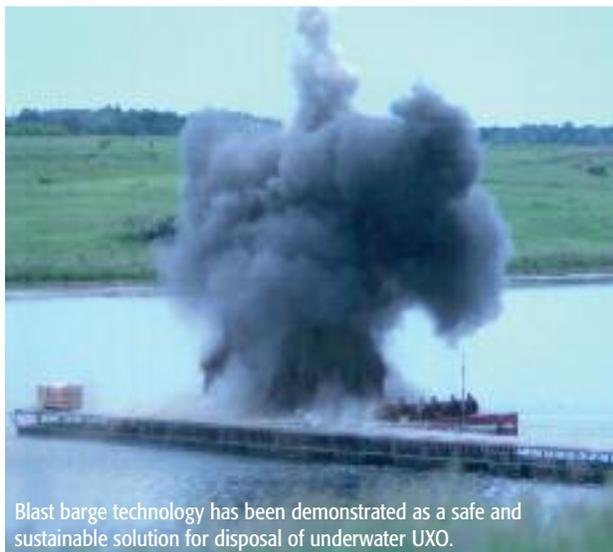
Blast barge technology has been demonstrated as a safe and sustainable solution for disposal of underwater UXO.
