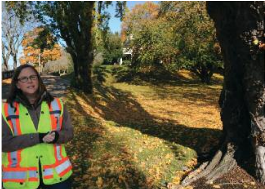
Amanda Bennett, Cultural Resources Specialist, NAVFAC Northwest, explains how 100-year-old Lombardy poplars, like this one, pose a potential danger to passing motorists and pedestrians during wind storms because branches have been known to break and fall.
