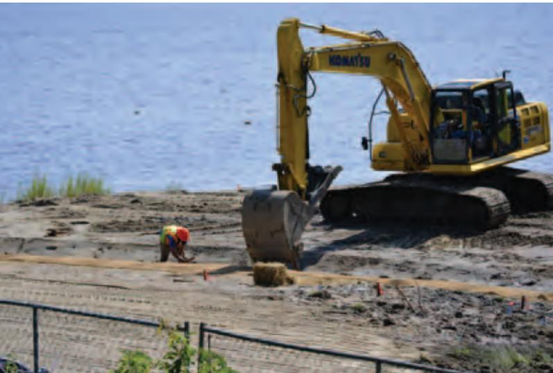
Members of a construction crew make final adjustments near the end of the initial construction stage of a stream restoration project at MCAS Cherry Point. Only weeks before, this piece of ground was the site of a dysfunctional concrete culvert that did a very poor job of routing stormwater runoff from an air station housing area to the Neuse River.
