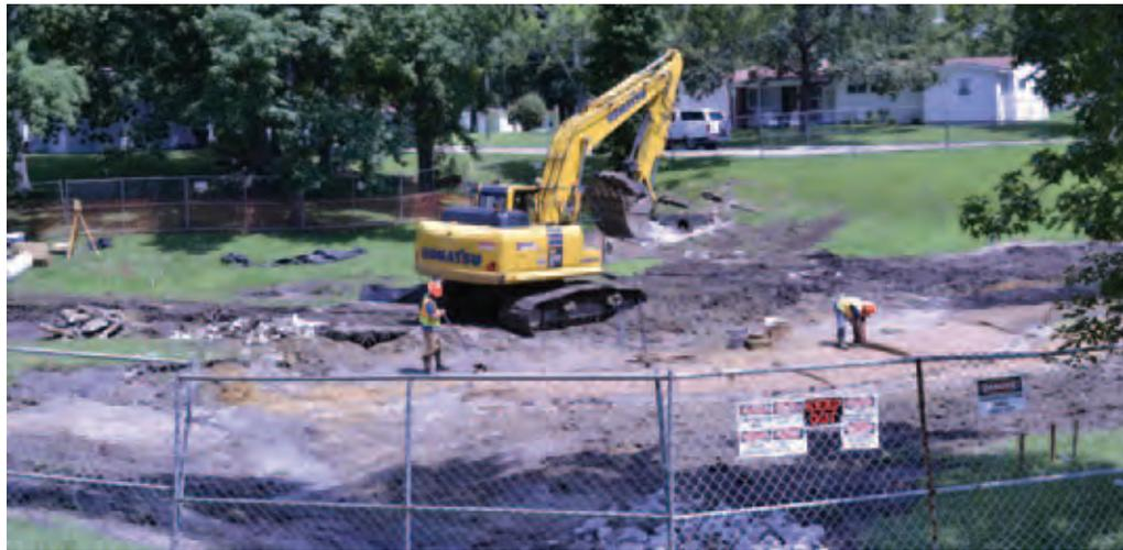
Members of a construction crew lay stabilizing mesh along the serpentine sides of a newly dug streambed during the initial construction stage of a stream restoration project at MCAS Cherry Point. The mesh will help control erosion of the stream’s banks until appropriate plant life is introduced to the stream’s riparian zone in later stages of the project.
