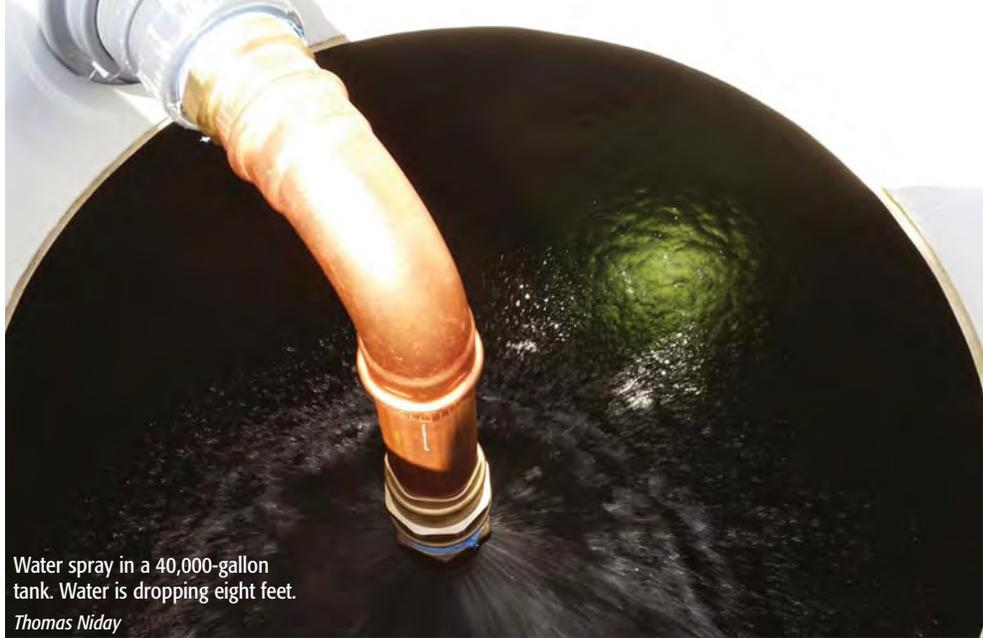
Water spray in a 40,000-gallon tank. Water is dropping eight feet.
