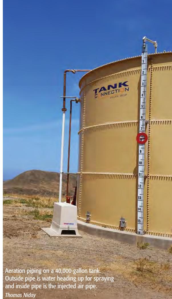
Aeration piping on a 40,000-gallon tank. Outside pipe is water heading up for spraying and inside pipe is the injected air pipe.
