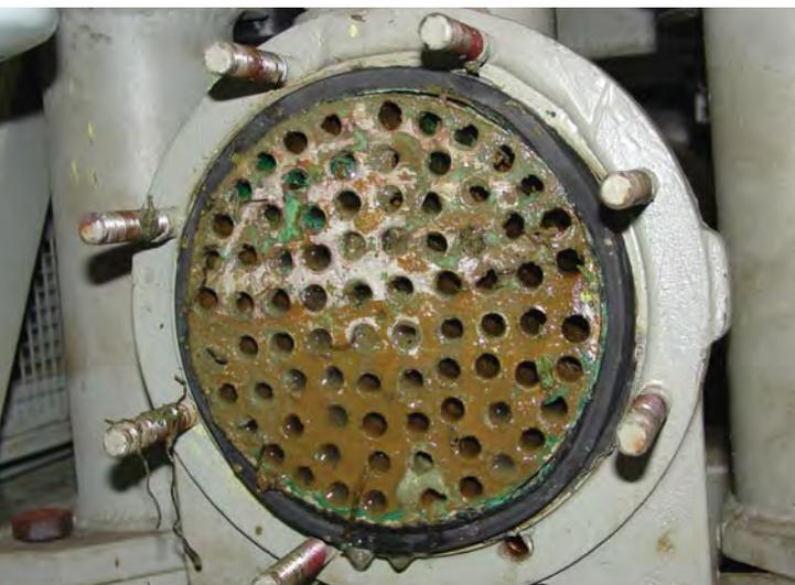
This photo of the internal heat exchanger tubing in LPAC No. 1 was taken at the conclusion of the demonstration of the I2 bubble technology, shows dirty, but not bio-fouled tubing.
