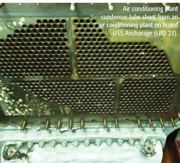
Air conditioning plant condenser tube sheet from an air conditioning plant on board USS Anchorage (LPD 23).
