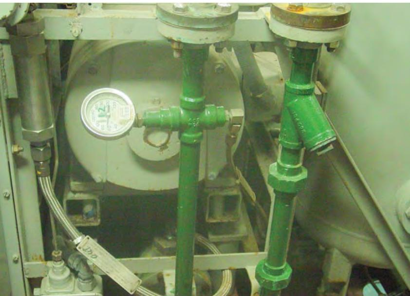
The number 1 LPAC heat exchanger onboard the SDTS.
