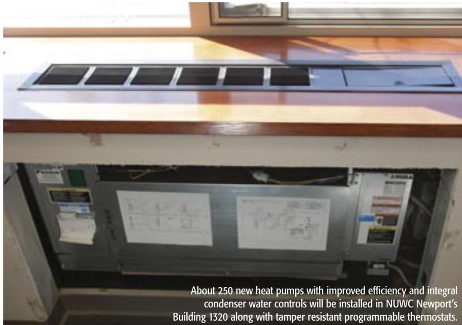
About 250 new heat pumps with improved efficiency and integral condenser water controls will be installed in NUWC Newport's Building 1320 along with tamper resistant programmable thermostats.
