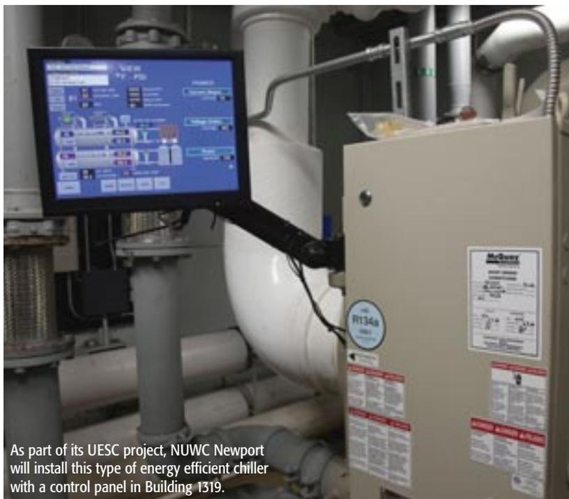
As part of its UESC project, NUWC Newport will install this type of energy efficient chiller with a control panel in Building 1319.
