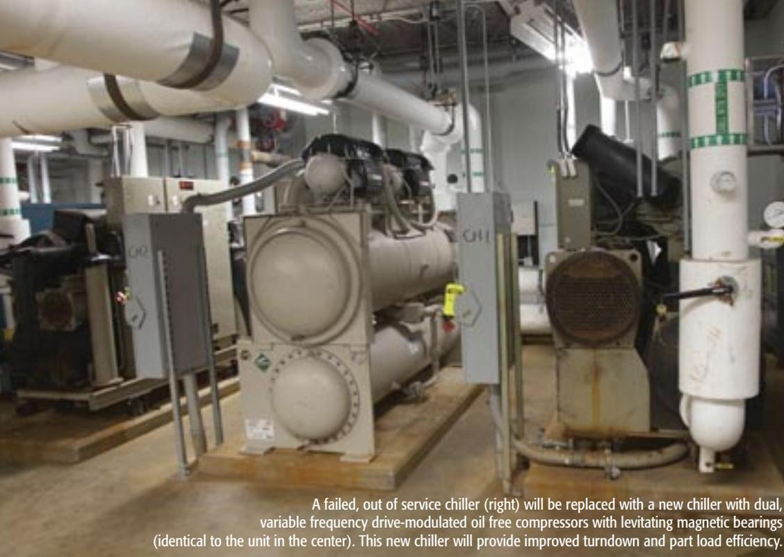
A failed, out of service chiller (right) will be replaced with a new chiller with dual, variable frequency drive-modulated oil free compressors with levitating magnetic bearings (identical to the unit in the center). This new chiller will provide improved turndown and part load efficiency.
