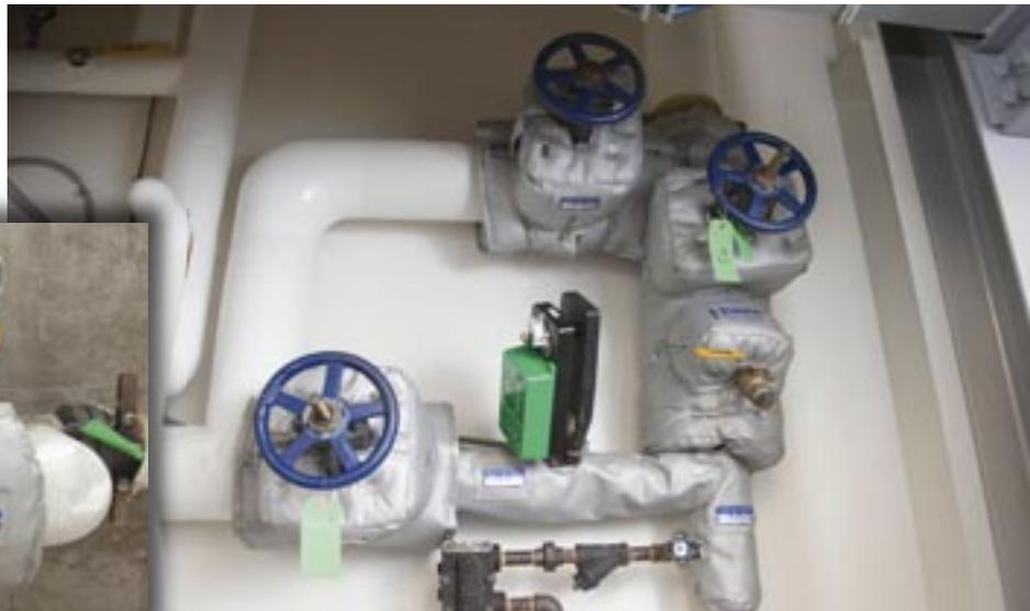
New insulated valve cover, steam trap and pipe insulation at NUWC Newport. The UESC project inventoried, tested, and tagged 520 steam traps, replaced 175 faulty steam traps, installed 350 feet of steam pipe insulation, and installed 302 insulated valve covers.
