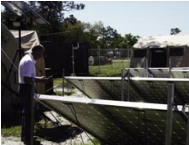
NSWC PCD engineer Dr. Lee Frye uses a hand held thermal imaging device to determine heat output levels inside the Warfare Center's expeditionary energy compound.
