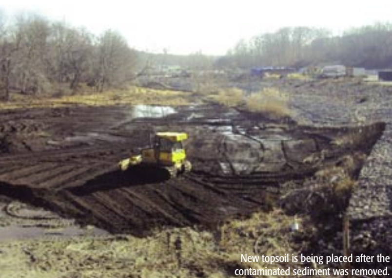
Contaminated sediment is removed from the wetland area.
