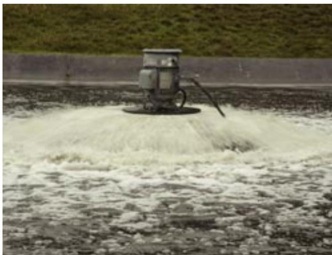
An aerator in the sewage lagoon is used to mix the water to facilitate microbial breakdown of the sludge as part of the primary phase of the wastewater treatment process.
