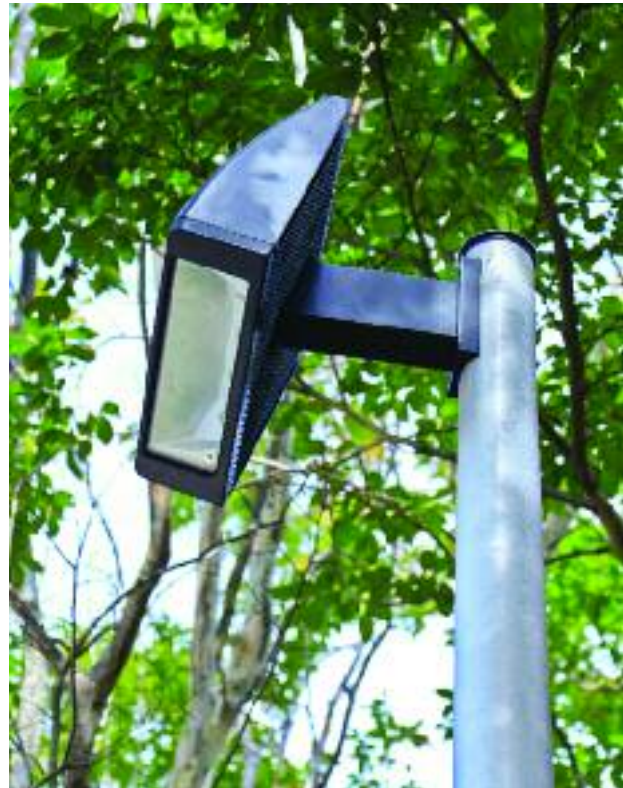
Photocells were mounted to all new LED lights at ATR to operate the lights from dusk until dawn only.
