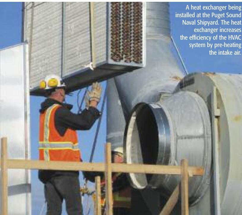
A heat exchanger being installed at the Puget Sound Naval Shipyard. The heat exchanger increases the efficiency of the HVAC system by pre-heating the intake air.
