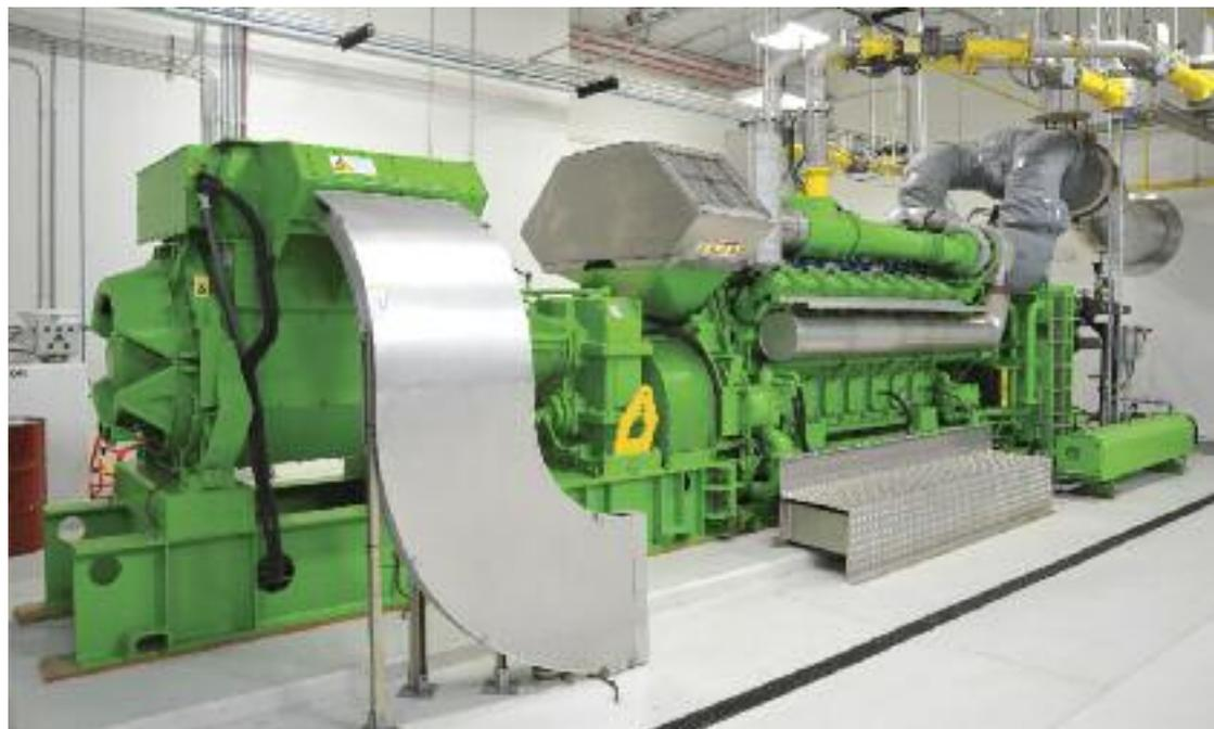
MCLB Albany's Landfill Gas-to-Energy generator produces 1.9 megawatts of renewable electric power and steam by burning landfill gas collected from the Gaissert Road Dougherty County Landfill. MCLB Albany, Chevron and local officials flipped the switch 23 September 2011. The new green technology is the first of its kind within the Department of the Navy.
