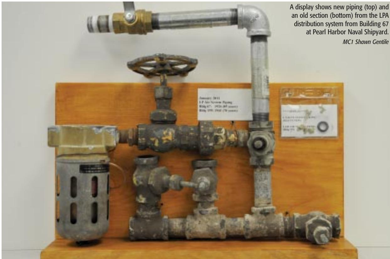
A display shows new piping (top) and an old section (bottom) from the LPA distribution system from Building 67 at Pearl Harbor Naval Shipyard.
