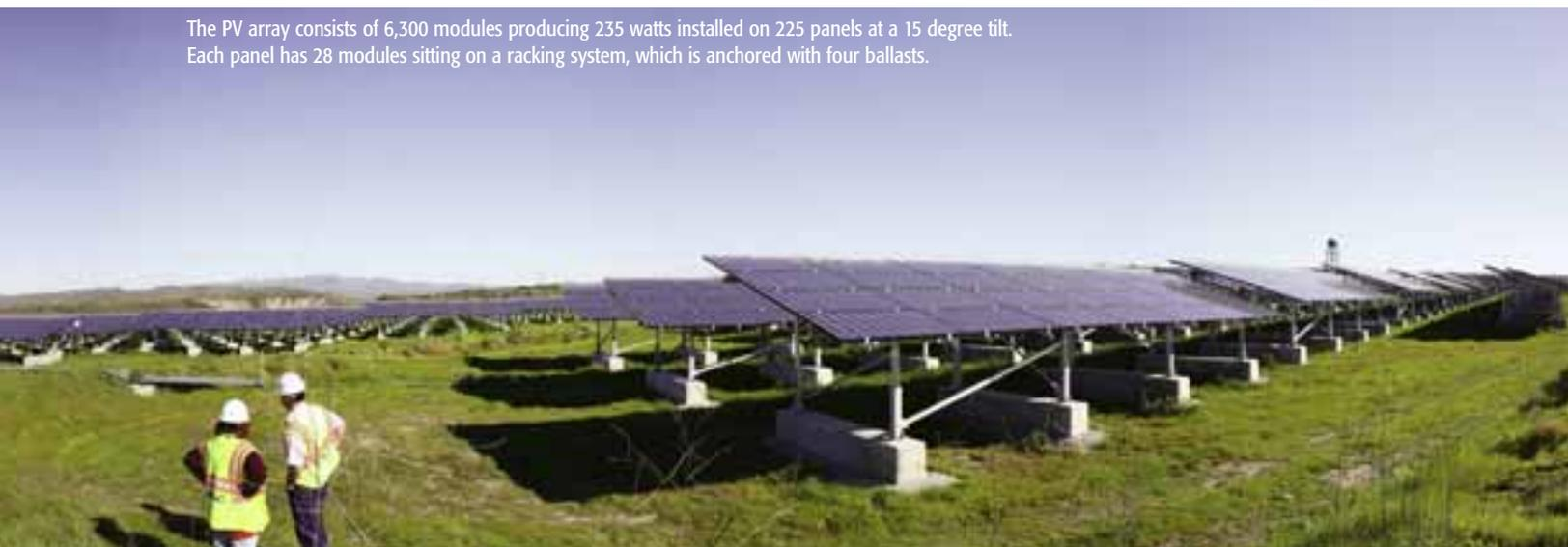
Marine Corps base. It is estimated that it will save the Marine Corps \$336,000 per year in electricity costs. This first PV array covers approximately five acres and includes 225 panels, each holding 28 modules for a total of 6,300 modules. The size of the system is 1.485 megawatts of direct current and will generate 2,400 megawatts per hour (MWH) annually, enough to power 400 homes. The project feeds into the Camp Pendleton electric grid.
