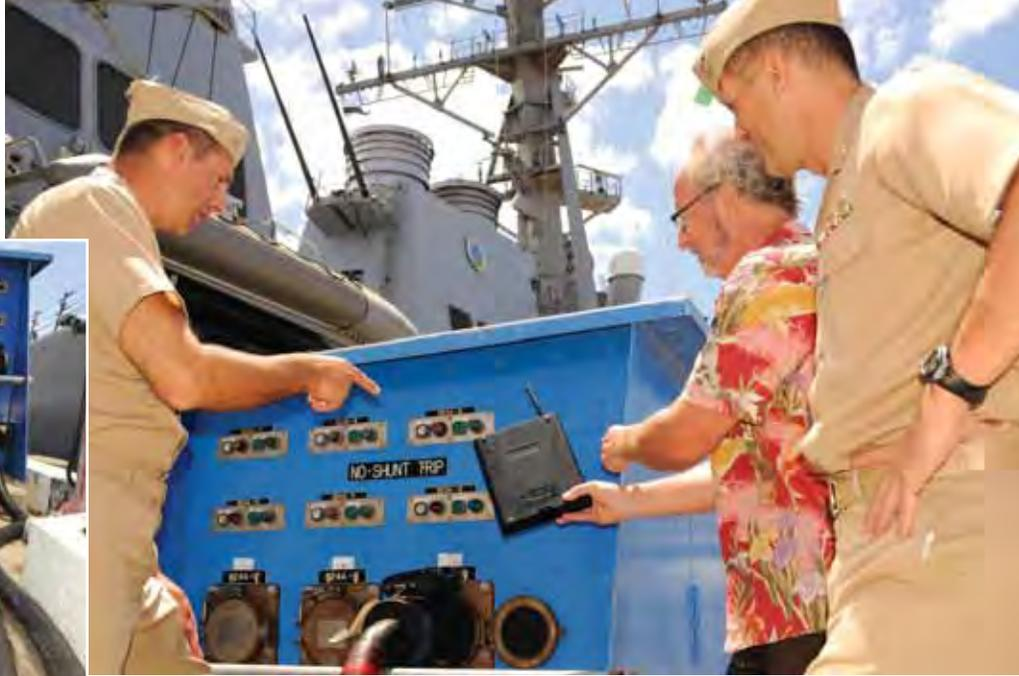
LEFT: Each capable of handling 400 amps, cables connect a ship to a "turtle back" shore-power source at Pearl Harbor.
