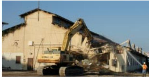
Building 146 is quickly crushed by a NAVFAC Hawaii equipment operator in February 2011. Comprised of mostly metals and wood, segregation of recyclable materials was executed to reduce construction debris transported to a local landfill.
