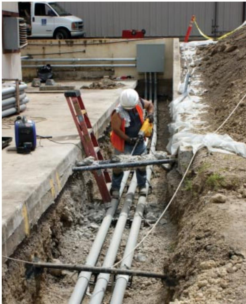
NAVFAC Hawaii utilities personnel relocated important electrical and compressed air lines out of warehouse Buildings 146 and 147 in September 2010, prior the buildings' demolition. Special trenches were dug to redirect power lines away from the two warehouses so that surrounding buildings would retain power after their demolition.
