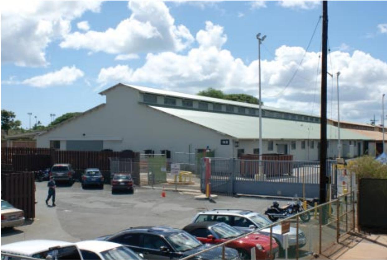
Renovations to Building 148, completed on 22 April 2010, retain historic aspects like wood windows, sliding doors, and light fixtures that were salvaged from Buildings 146 and 147 as well as new corrugated roofing and siding that were installed and painted to mimic the original look of the warehouse. The building is now being used as storage and office space by commands at Pearl Harbor.
