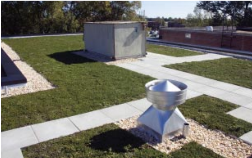
The newly installed green roof on Building A-50 at NS Norfolk.
