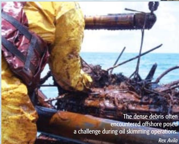
The dense debris often encountered offshore posed a challenge during oil skimming operations.
