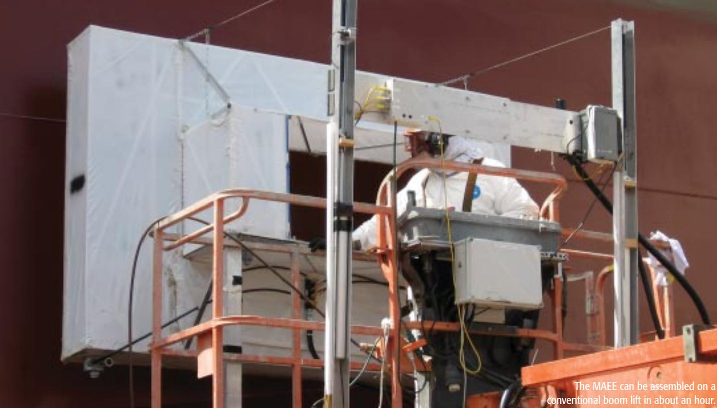
The MAEE can be assembled on a conventional boom lift in about an hour.
